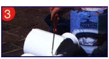
**3.** Connect the PoolSkim elbow from the body of the PoolSkim to the union (ring nut, o-ring, and stub). See picture to view elbow placements for various pool inlet (return jet) locations. If used in the connection process, the enclosed PVC 7 inch pipe can be cut for a customized fit. Next, use the stainless steel screws to fasten the elbow connections.
